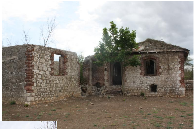
Plate 7 & 8. Showing trees in wall crevices on outbuildings
