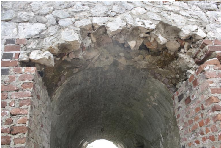
Plate 11. Showing arches without support beam
