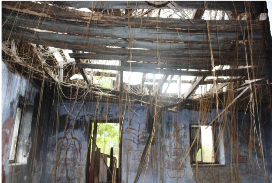
Plate 9. Showing trees in wall crevices
