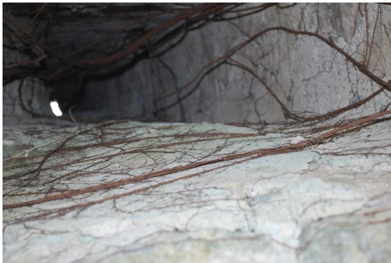
Plate 15. Showing roots growing from the top of the of the structure
