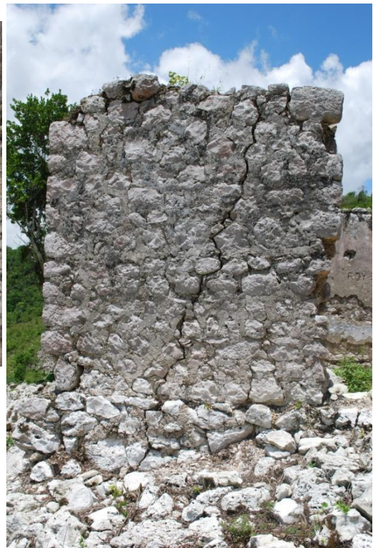
Plate 19. Showing large crack in a wall of the structure
