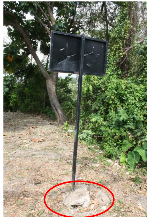
Plate 6. Rear of No Trespassing sign showing puncture holes and dislodgement
