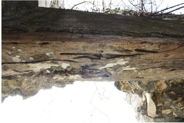
Plate 15. Showing deteriorating wood
