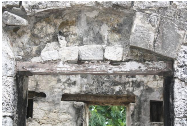
Plate 17 &18 Showing stones breaking away
