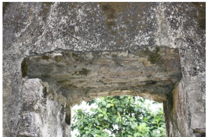
Plate 14. Showing window with missing support
