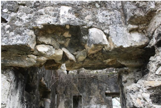
Plate 17 &18 Showing stones breaking away
