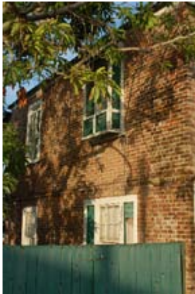
This early 19th century Flemish bond brick house was red washed to look like common red brick buildings.
