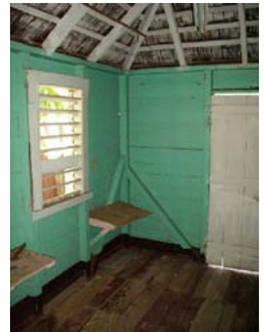
The inside of this small board house also has an exposed roof system to promote greater air circulation.
