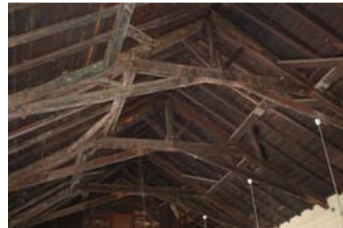
An exposed king post truss roof framing system.
