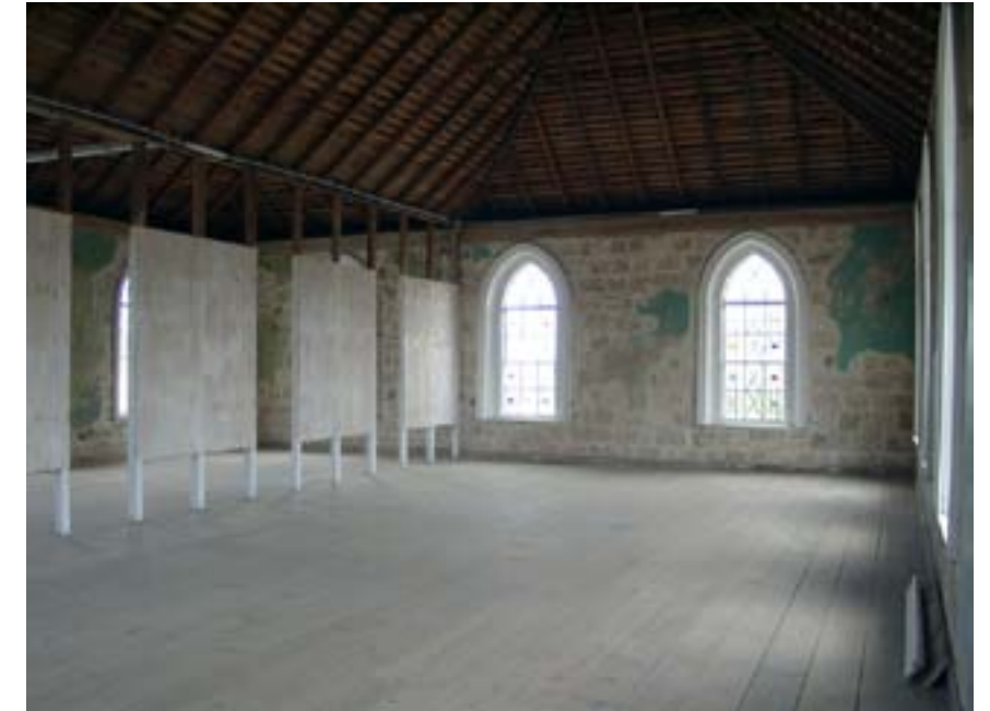
The roof framing system on the interior of the Baptist Manse (c. 1798) is left completely exposed to help cool the inside.
