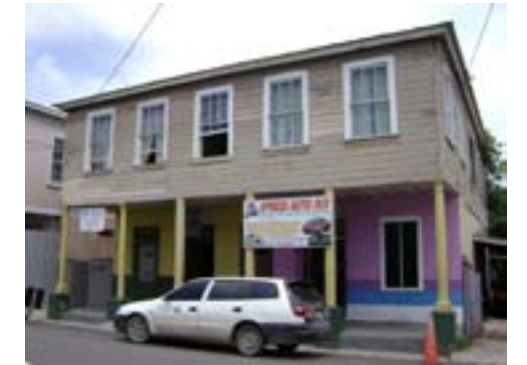
This commercial building on Market Street possesses a masonry ground floor and timber frame second story.
