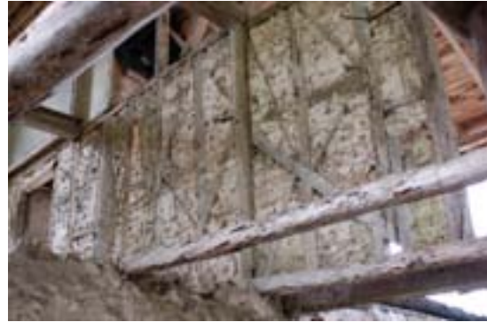
The image above shows a typical nogged building.
