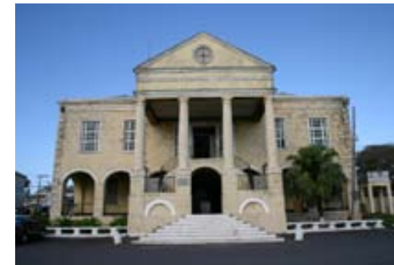
The Falmouth Courthouse is constructed of local cut block limestone.
