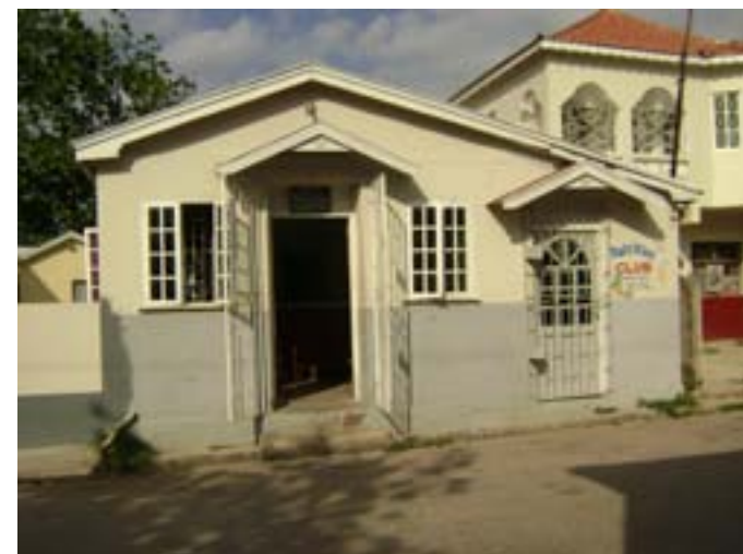
Left: Cast concrete and concrete block are appropriate materials for new construction in the Falmouth Historic District, but should be parged and painted in an appropriate way. Right: Concrete block walls as shown in this image should not be left exposed.
