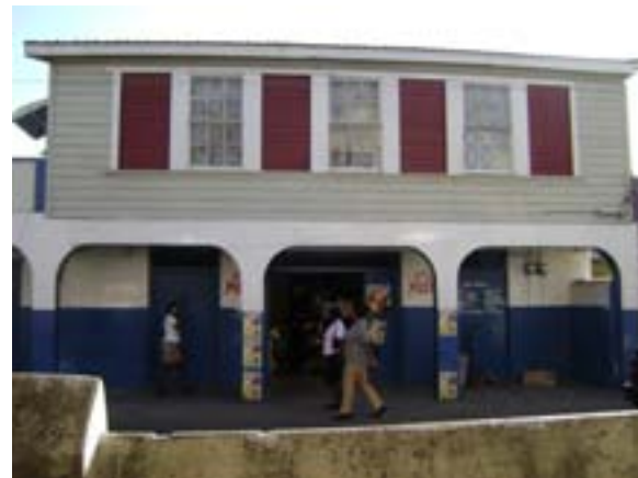
These commercial buildings on Market Street show how the first floor is often recessed in order to provide a shady walking area for pedestrians. This method of construction also helps articulate the bays of a structure and provide visual interest.
