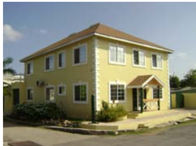
Above: A newly constructed fence on a historic home appropriately utilizes detail and decoration consistent with the historic district. Below: A newly constructed home employs details consistent with Falmouth's historic fabric, including quoins and a decorative gable roof over the entrance.
