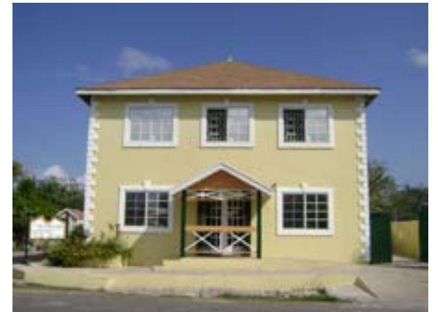
Above: Often the lower portion of a house will be painted grey or dark red to distinguish the foundation from the rest of the structure. Below: A new concrete home constructed in the historic district that was appropriately parged and painted.
