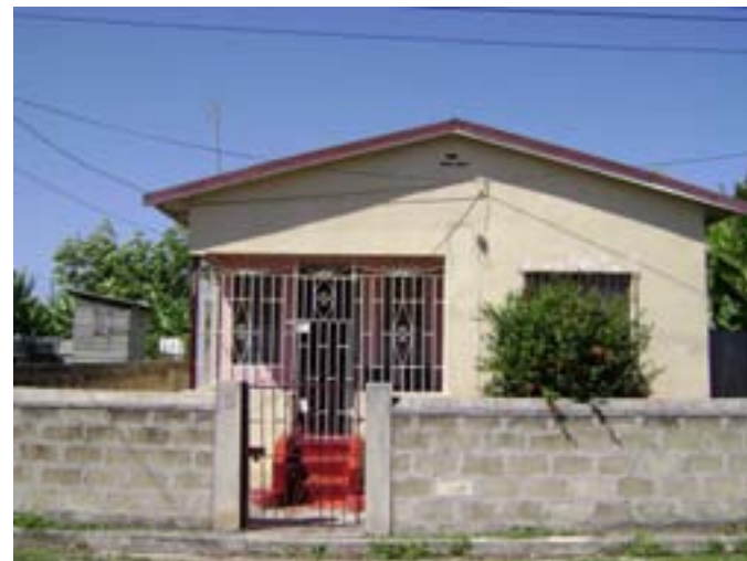
Left: Cast concrete and concrete block are appropriate materials for new construction in the Falmouth Historic District, but should be parged and painted in an appropriate way. Right: Concrete block walls as shown in this image should not be left exposed.
