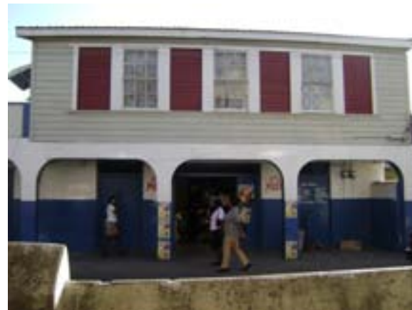
These commercial buildings on Market Street show how the first floor is often recessed in order to provide a shady walking area for pedestrians. This method of construction also helps articulate the bays of a structure and provide visual interest.
