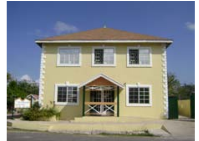
Above: Often the lower portion of a house will be painted grey or dark red to distinguish the foundation from the rest of the structure. Below: A new concrete home constructed in the historic district that was appropriately parged and painted.
